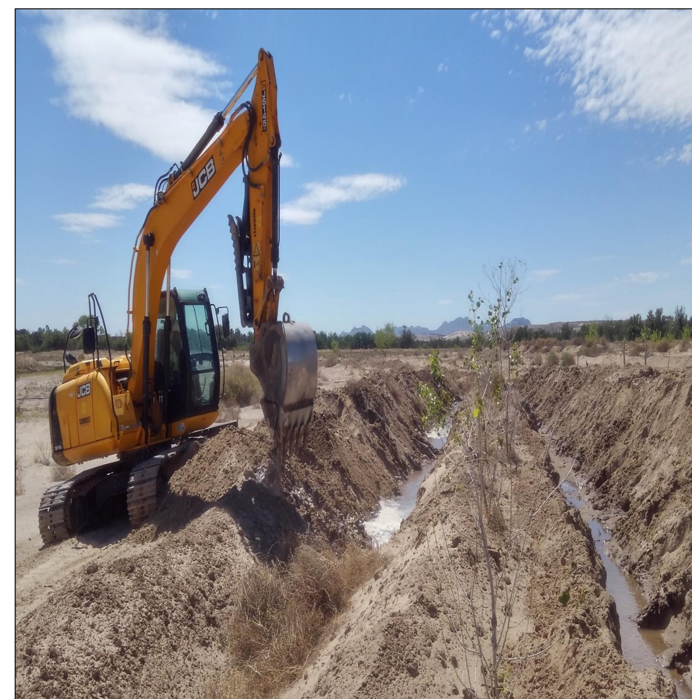
Figure 1. Excavator digging trenches at ReNUWIt Sunland Park Test-Bed.
