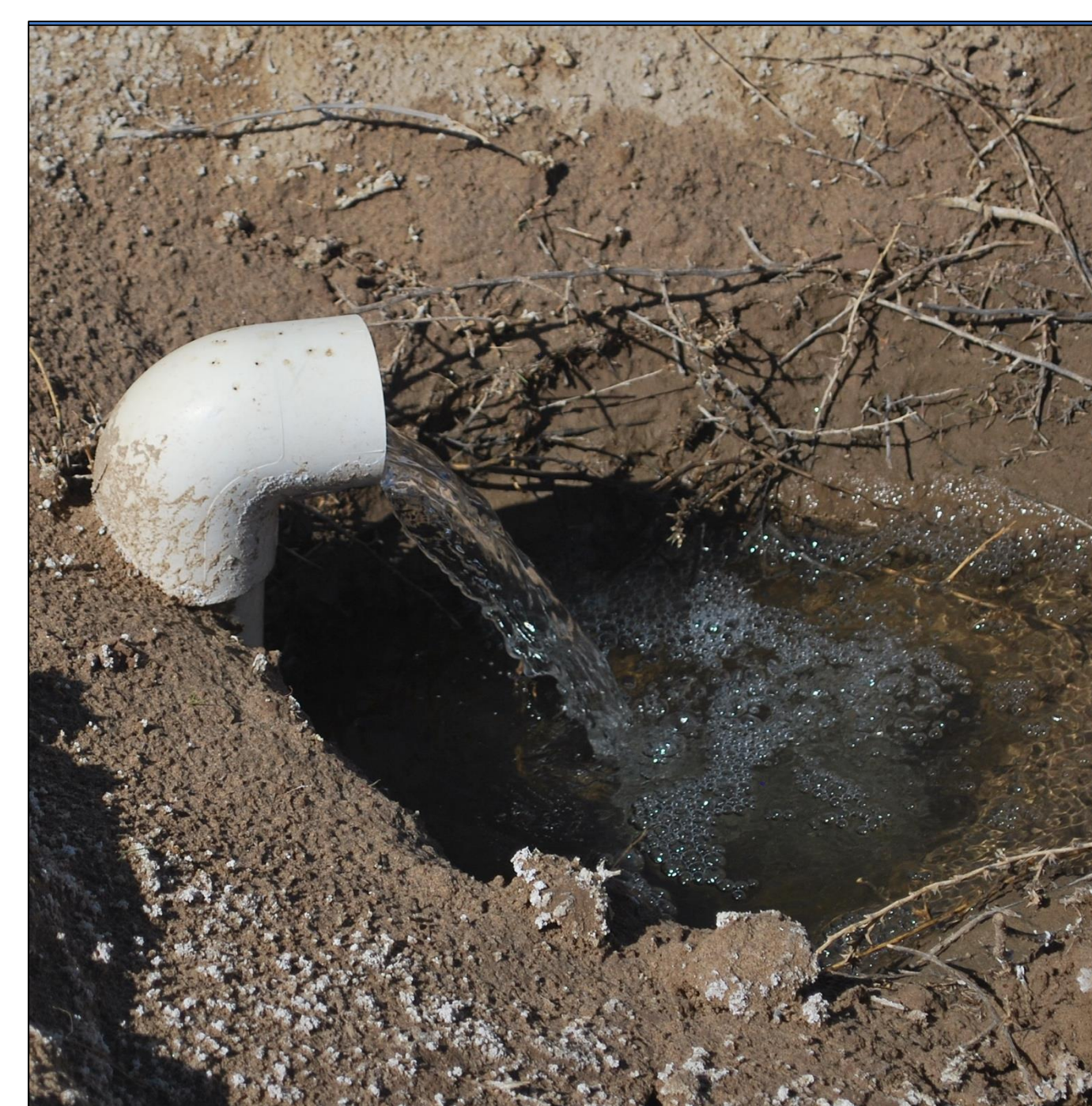
Figure 6. Water pumped from Diez Lagos canal, into trench.
