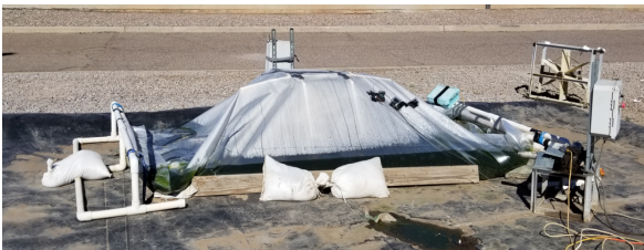
Figure 1: One of the two 700L pilot scale algal reactors of the POWER system deployed at the Las Cruces wastewater treatment plant
