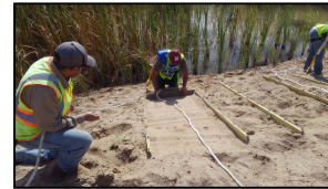
Figure 2. Installation of experimental plots in the embankment.
