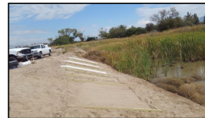
Figure 4. Set up of experimental plots on the embankment (3ft x 8 ft.) at ReNUWIt testbed site.
