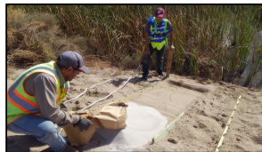
Figure 3. Pouring zeolite in designated experimental plots (3 in. layer).
